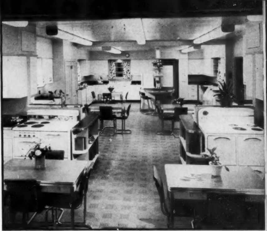
AFTER What a difference: five kitchen units, fully equipped with modern ranges, refrigerators, electric sinks and other appliances; the automatic home laundry installation; the informal snack bar. Students grin when they walk into this classroom!
